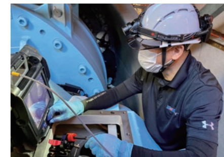
Wind power plant/borescope inspection
